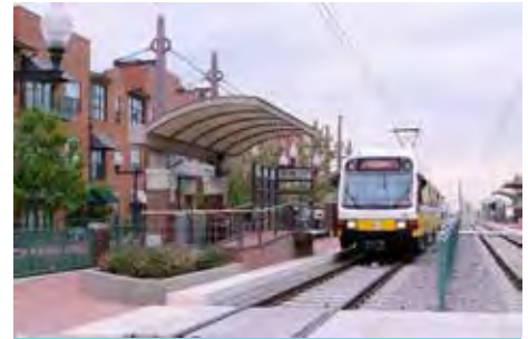
DART Rail Transit Station
