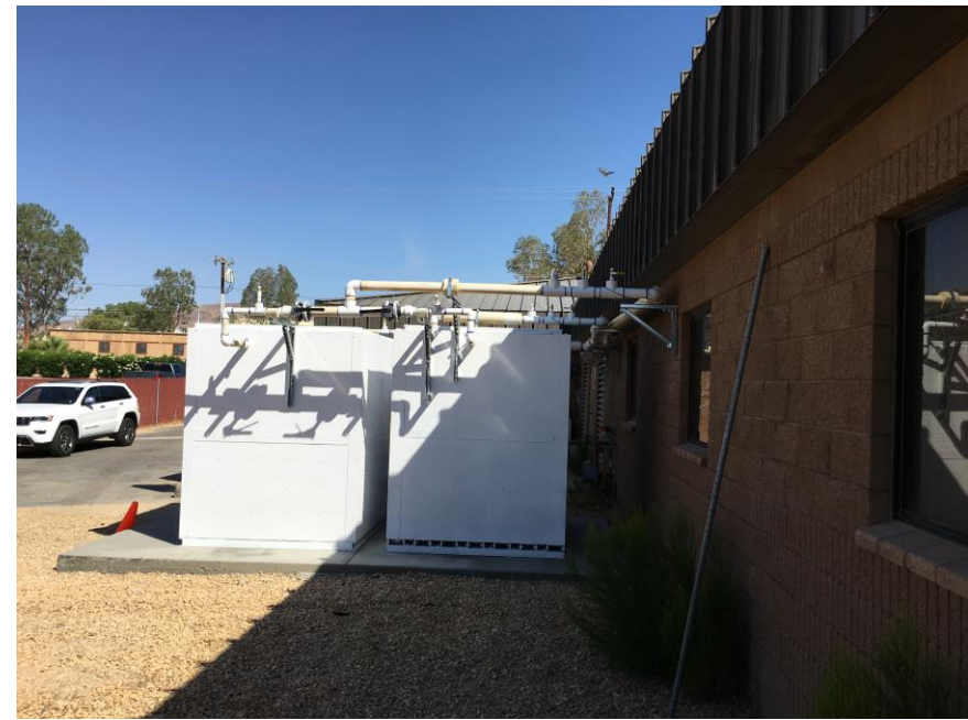
PhaseStor Install, rear service yard, B1020
