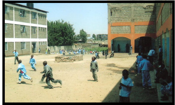
Future Dormitory—Kitchen/Dining Hall Building and playground.
