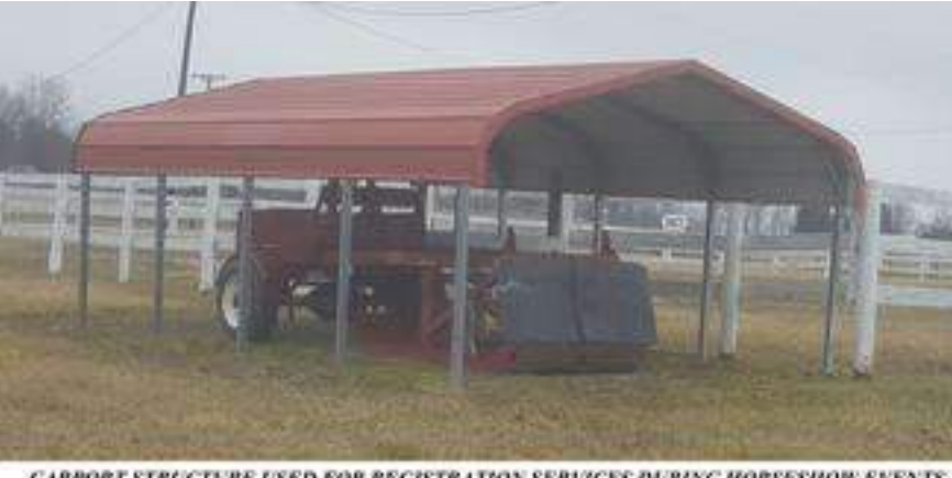
CARPORT STRUCTURE USED FOR REGISTRATION SERVICES DURING HORSESHOW EVENTS
