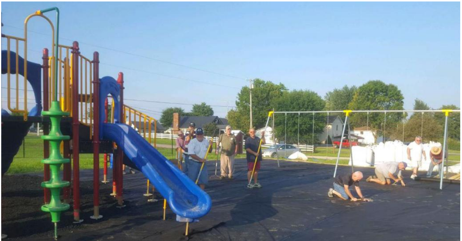
Tollesboro Lions Club members present for a “work-night” installing filter fabric and rubber mulch.
