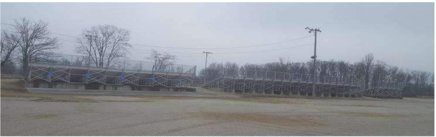
BACK SIDE OF PERMANENT BLEACHERS
