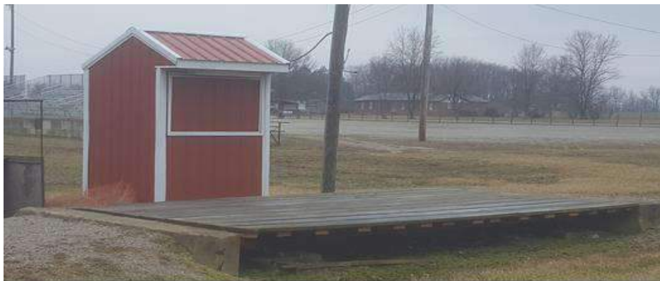
On-Site Scales and Scale House for weighing Tractors for Tug Tractor Pull and other Events
