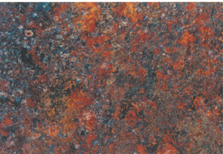
INITIAL CONDITION D
