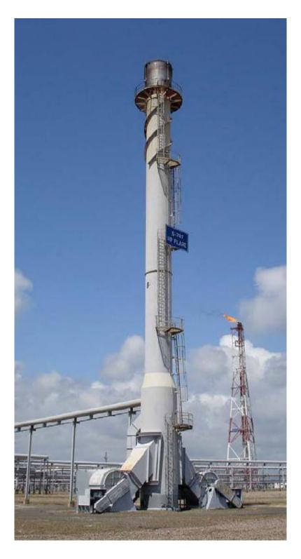
A gas flare, alternatively known as a flare stack or tower is used to eliminate waste gas which is otherwise not feasible to use or transport. They also act as safety systems for non-waste gas and is released via pressure relief valve when needed to ease the strain on equipment
