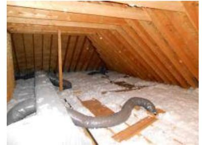
*Roof Framing:* A rafter system is installed in the attic cavity to support the roof decking.
