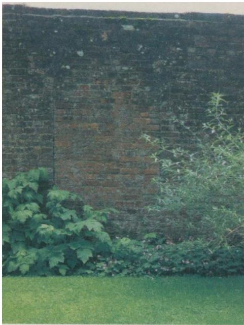
Bricked up door of the walled garden at Maytham Hall.
