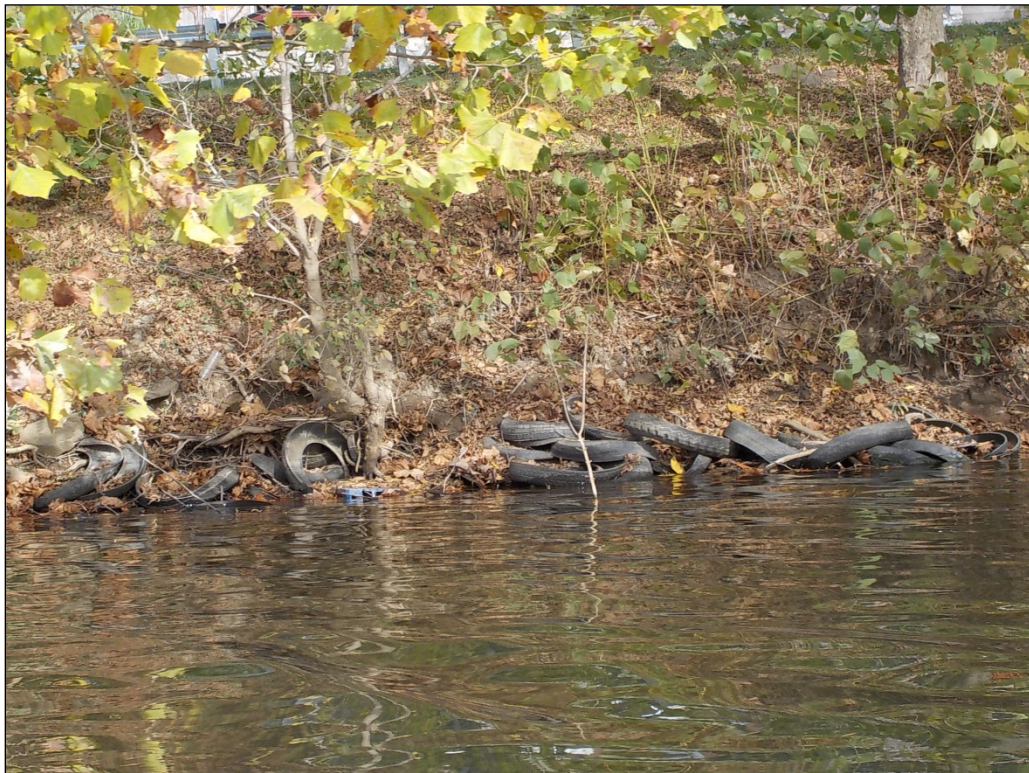
Photograph 20 – NE riverbank stabilization using waste tires, view NE
