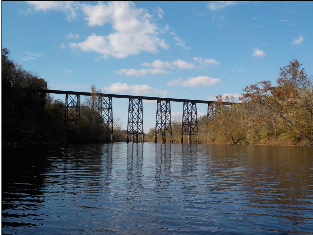
Photograph 9 – Existing railroad bridge across Woodruff Island, view NW
