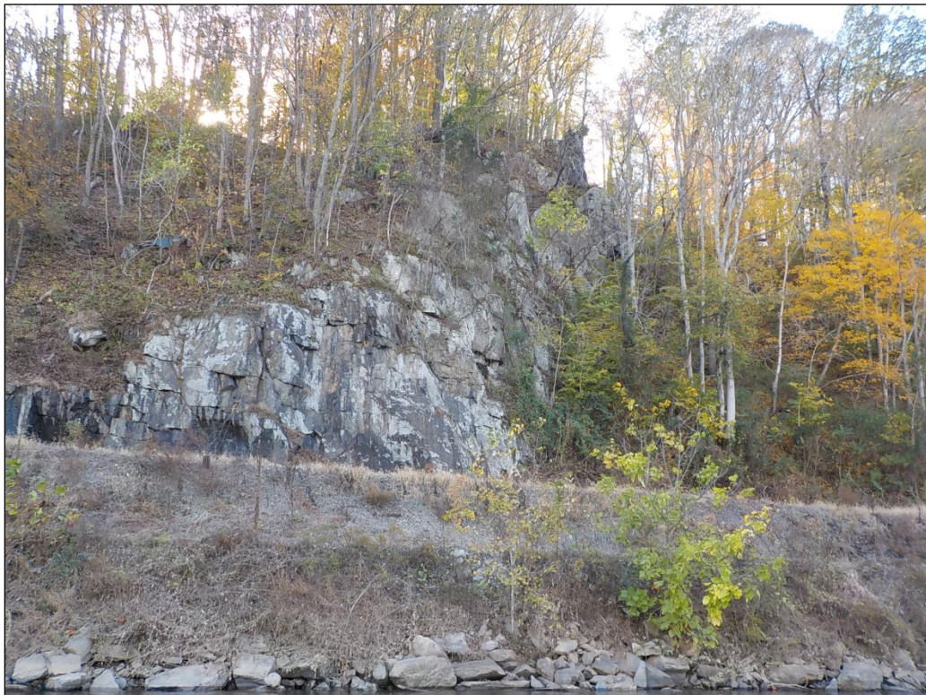
Photograph 10 – Typical SW riverbank, with railroad and >10' high riprap stabilization (view W)
