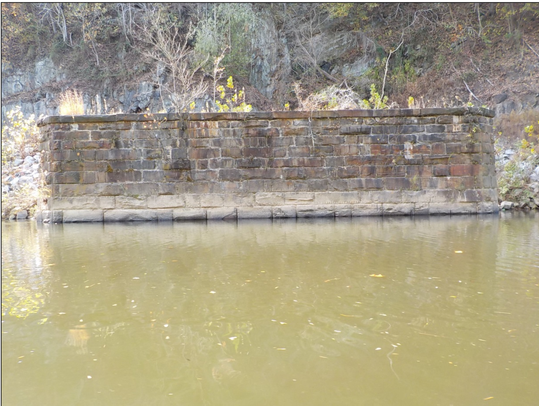
Photograph 8 – Relic stone railroad bridge pier, view SW
