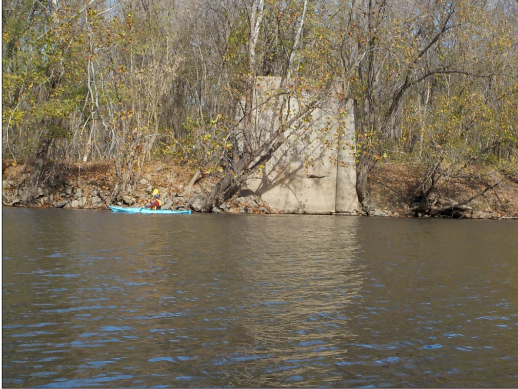
Photograph 7 – Bridge abutment (?) / structure on Treasure Island, view E
