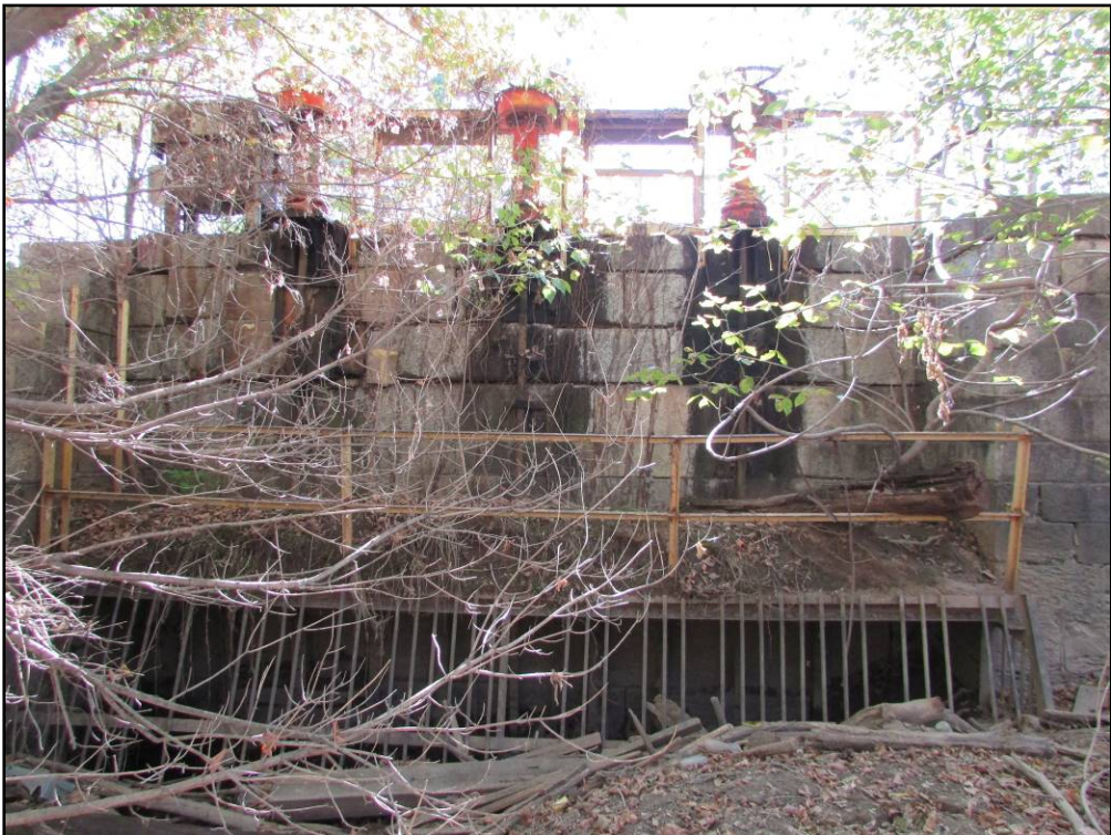
Figure 5. Water Works Gate and Locks, view to the East.
