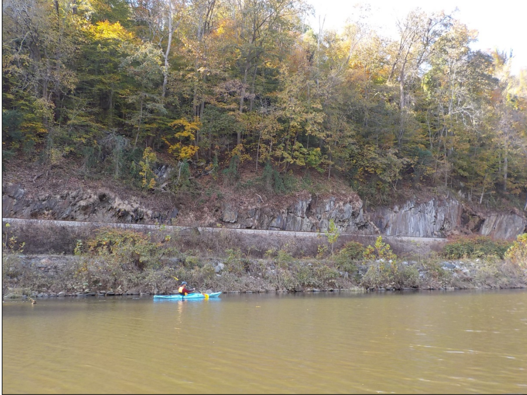
Photograph 3 – Typical southwestern riverbank (note railroad riprap), view SW
