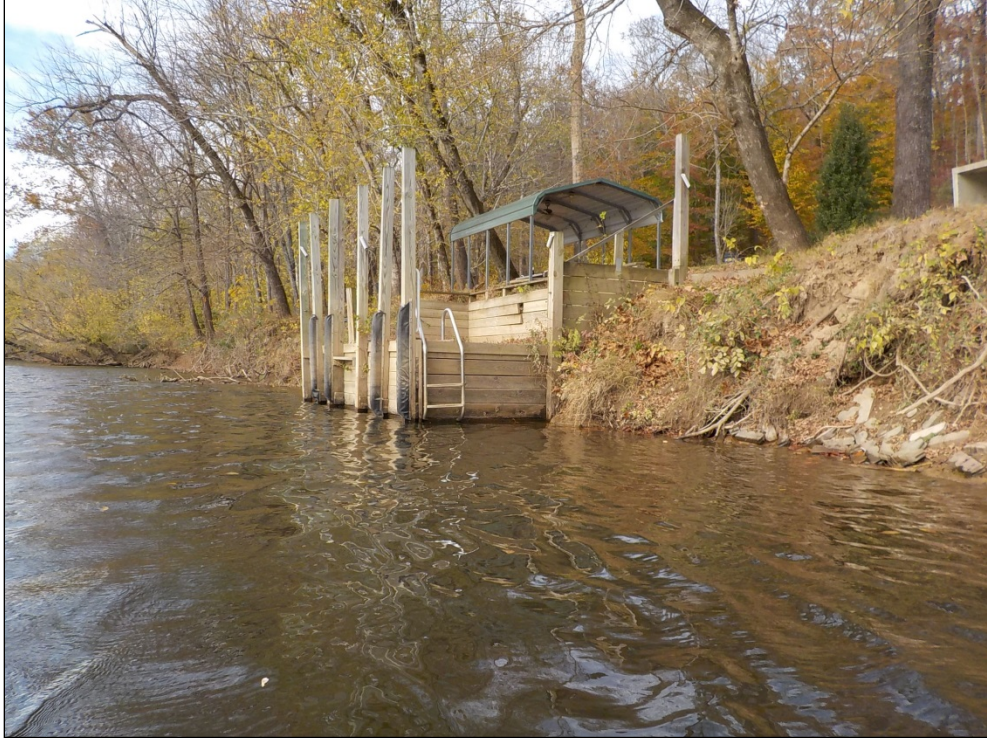
Photograph 13 – Typical NE riverbank development and boat dock, view N
