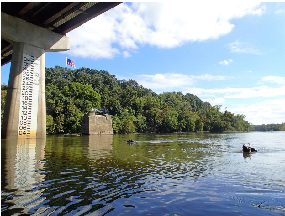
Snorkeling run habitat under John Lynch Bridge-tailrace reach
