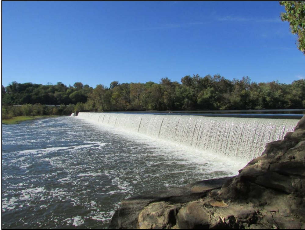
Figure 9. James River Dam, view to the south.
