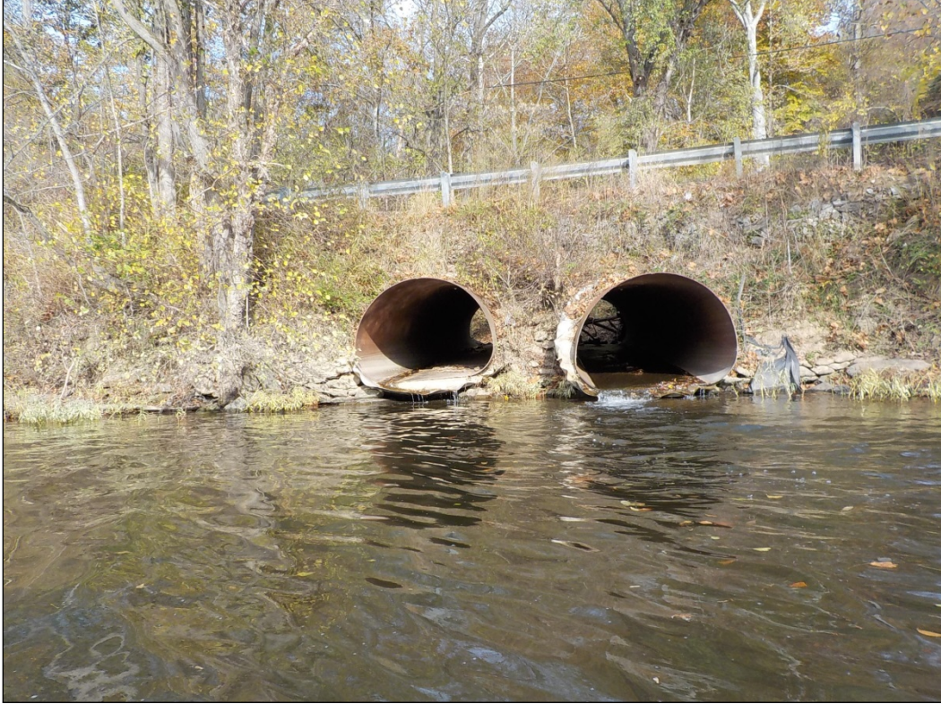
Photograph 19 – Roadway along NE riverbank (note >8' riverbank height), view NE
