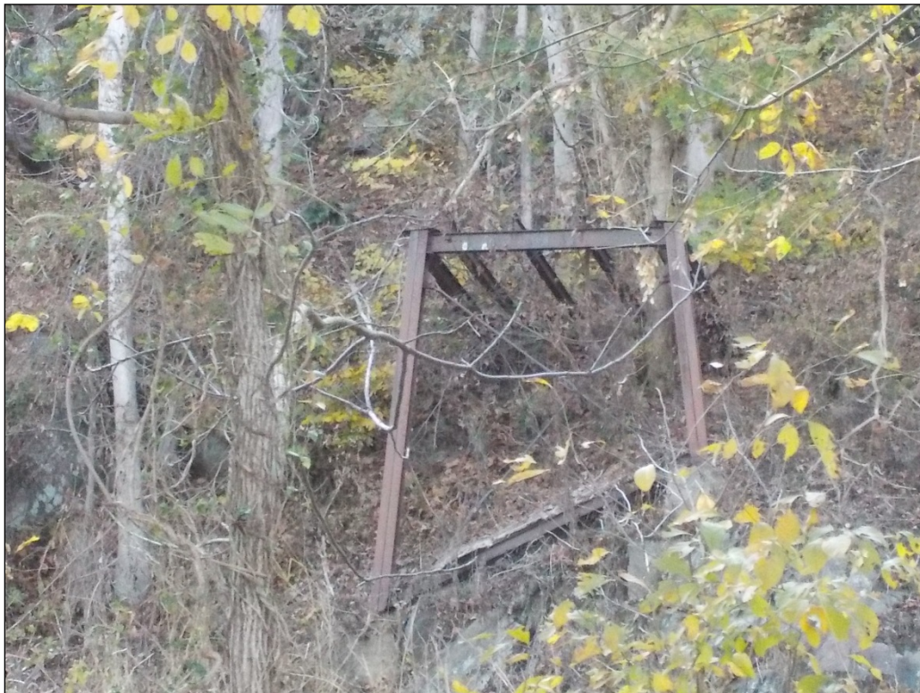
Photograph 6 – Relic bridge abutment on SW riverbank (view NW)
