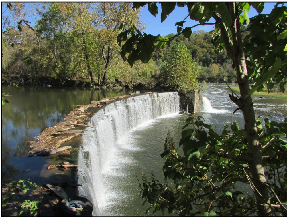
Figure 3. Water Works Dam, view to the North.
