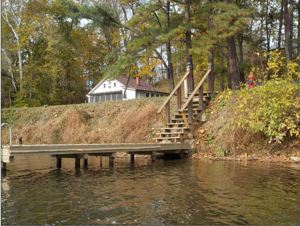
Photograph 15 – Typical NE riverbank pier/dock (note 10' riverbank), view N
