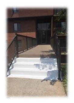
Northern Waterproofing & Restoration Co., Inc. was called-in by Westover Companies, in order to restore and preserve their existing concrete balconies as well as, all concrete pedestrian bridges. Following jobsite mobilization, NWR removed all failed coating and/or deteriorated concrete throughout, and replaced all railings with new powder coated aluminum. Following the concrete repairs, NWR applied a new ure-
