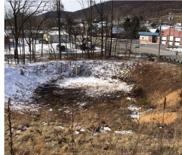
Commercial development stormwater management facility.
