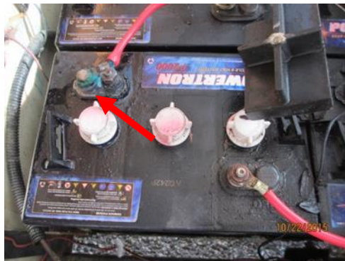
Previous Corrosion
