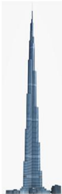
Microwave Receive Site at Burj Khalifa
