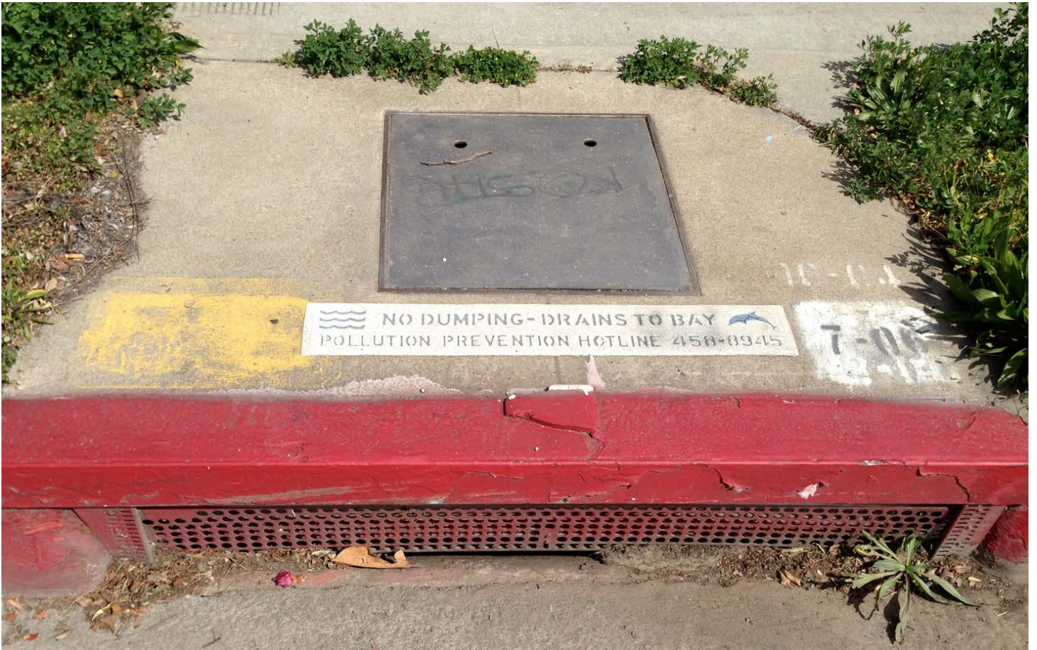
Full capture device in the City of Los Angeles. (Photo taken by Stephen Joseph in Brentwood on 3-2-13)
