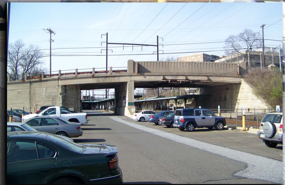
Existing Site Condition
