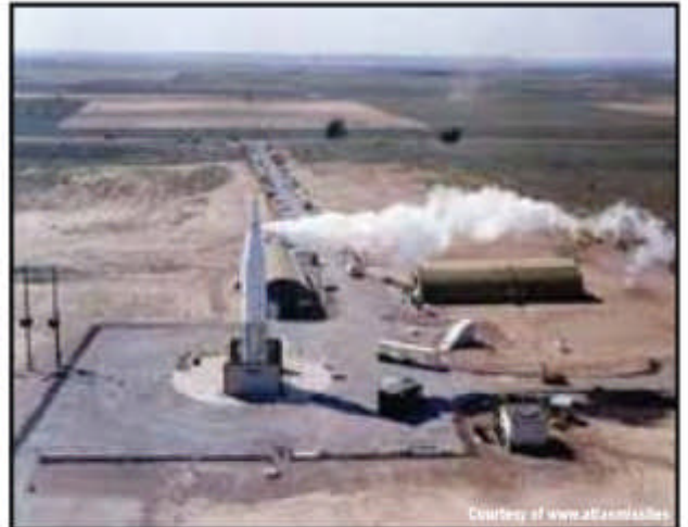
Top: Jeff Flaningam walks through the tunnel connecting the missile silo to the command center. Left: Three images were merged to be able to see the inside of the top of the silo down to the water. Above: Seen is an Atlas F missile at Willow, Okla., which was Site 11 of the 577th SMS based at Altus Air Force Base.
