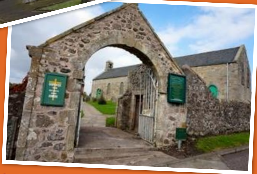
Building at Kinglassie
