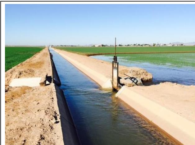
Figure 3.6a Concrete Lined Ditch
