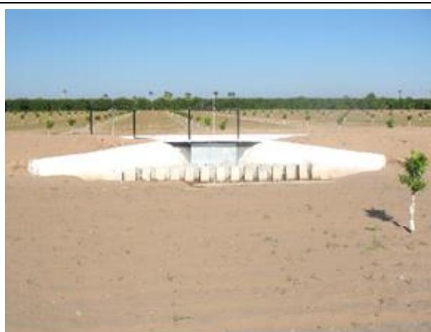
Figure 3.6b High Flow Irrigation Turnouts
