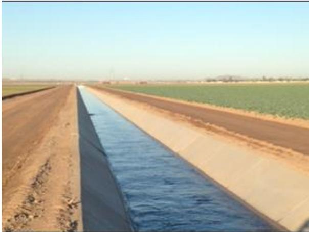
Figure 2.1 Concrete Lined Canal
