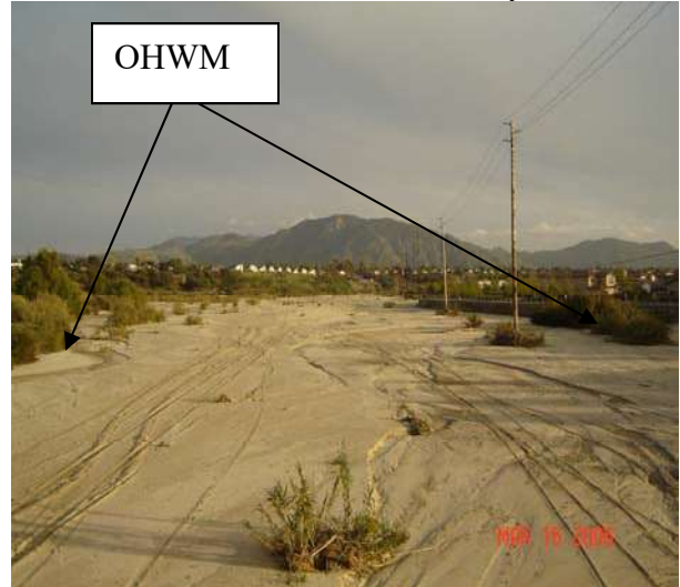
Photo 21. Soft-bottom intermittent tributary with a flood control levee, Ventura County, CA.
