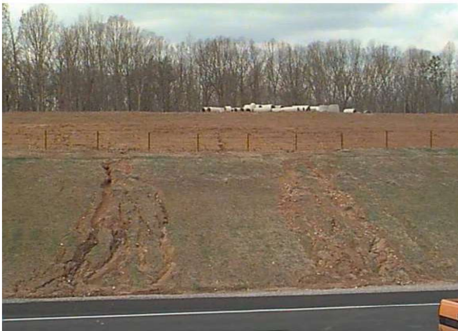
Photo 60. These erosional features are small channels eroded into the soil surface by runoff.
