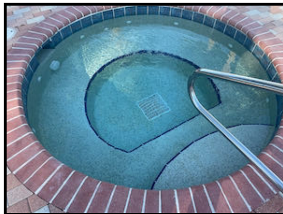
Spa Area With No Indications of Damage
