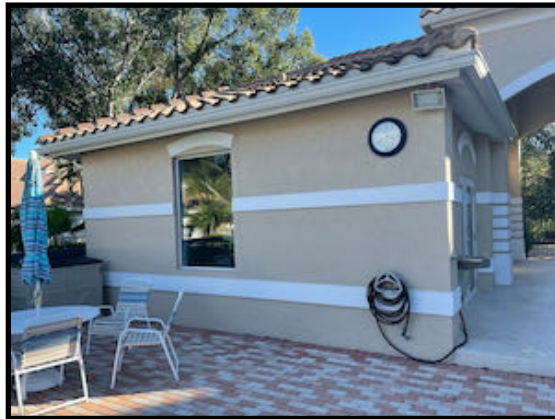
No Signs of Lightning Damage to Clubhouse
