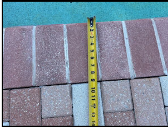
Measuring Coping at Edge of Pool
