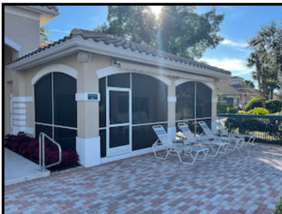
No Signs of Lightning Damage to Clubhouse
