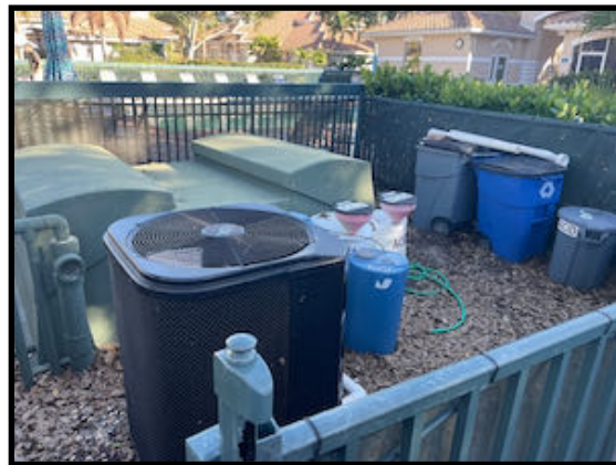
No Indications of Damage to Pool Equipment
