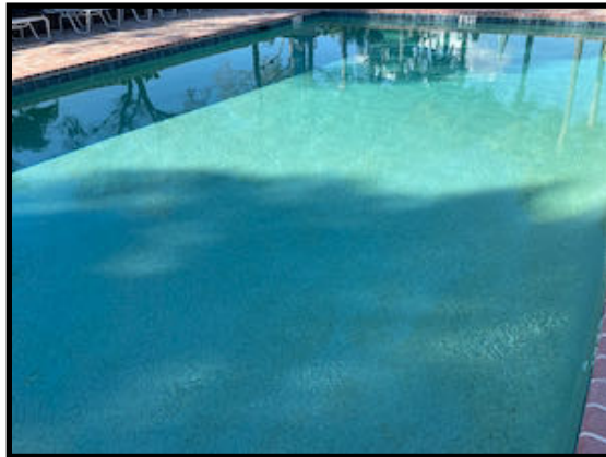
View Inside Swimming Pool
