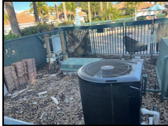
No Indications of Damage to Pool Equipment
