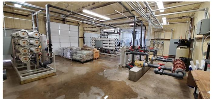
Raw water from the wells is delivered to a 250,000-gallon tank on the RWC site and is subsequently treated for removal of arsenic, nitrate, fluoride, total dissolved solids (TDS) and any other potential contaminants ensuring it meets the strict safe drinking water standards. The water is then disinfected with sodium hypochlorite prior to storage in a 250,000-gallon Potable Water Storage tank located on the RWC site.
