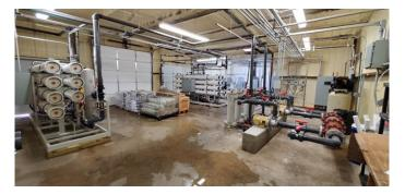
Raw water from the wells is delivered to a 250,000-gallon tank on the RWC site and is subsequently treated for removal of arsenic, nitrate, fluoride, total
