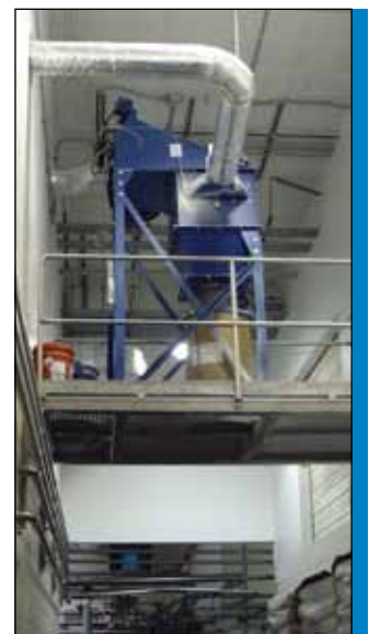
CPV-3 Powdered milk dust in cheese factory (1200 cfm)
