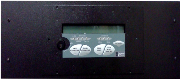
Figure 1 FCI KDU Retrofit
