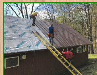
A new metal roof was put on the Joe Boyd Boys' Dormitory.
