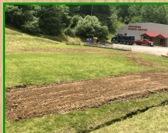
Dirt added to crown the ballfield to make it level.
