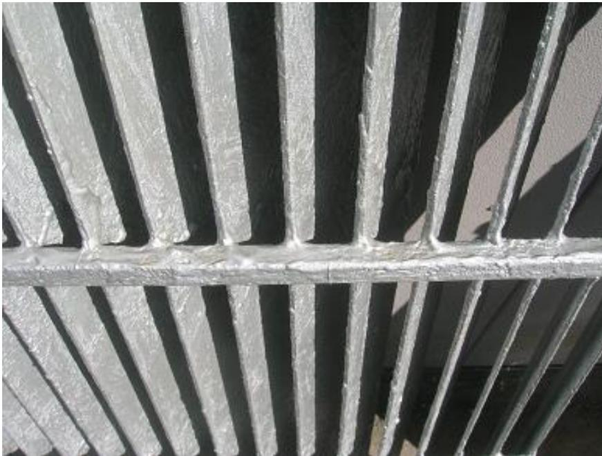
A close-up image of the louver array above shows that the paint was applied thick and uneven in areas, giving the louvers a slightly rough, patchy and lumpy texture.
