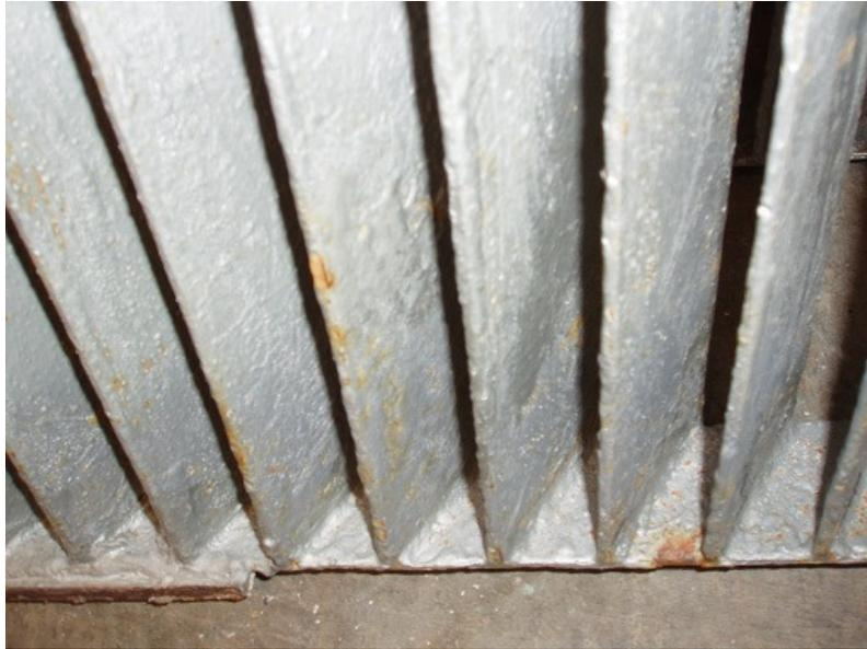
Currently, there are also a few places on the louver arrays where small sections of paint are peeling off as shown on middle louver blade in the picture below. Unfortunately, the image is slightly out of focus.
