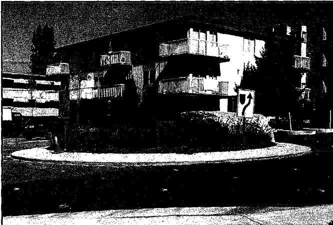
Traffic circles work to slow traffic in residential neighborhoods. This Vancouver traffic circle was built by the city and planted by local residents
