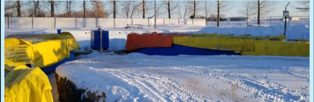
Picture shows the expansion walls have been installed.
