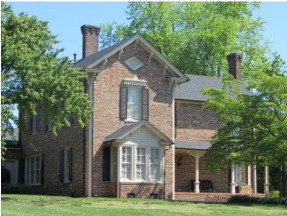
Figure 75. NCDOT Survey #11, Joseph Bason Whitsett House (GF-2148), 7241 Burlington Road, Guilford County, main house looking northeast showing modern brick veneer.
