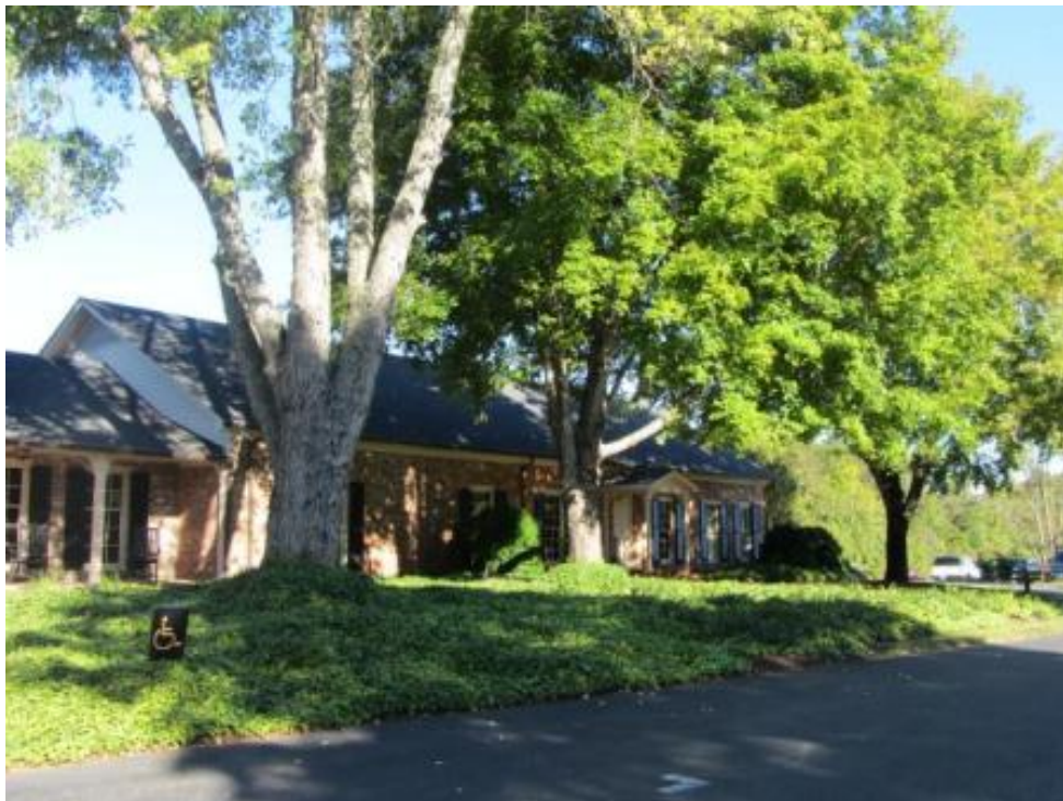
Figure 77. NCDOT Survey #11, Joseph Bason Whitsett House (GF-2148), 7241 Burlington Road, Guilford County, north section of the rear addition to the house built in the late 1980s, looking northwest.
