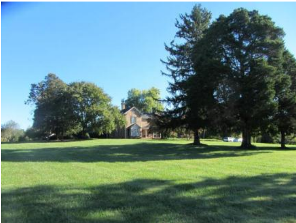
Figure 73. NCDOT Survey #11, Joseph Bason Whitsett House (GF-2148), 7241 Burlington Road, Guilford County, main house and extensively landscaped grounds looking north from US 70.
