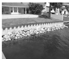
Vinyl Seawall with Rip Rap
