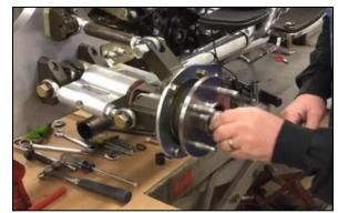
Step 44 Install the Wheel Flange/Hub (part #1304) with lug nut bolts into the Outside Carrier (part #1314), using one 7/8" Flat Washer (part #1324) and one 7/8" Locking Nut (part #1326)
