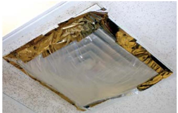
⚡ An operational issue identified during the Assessment phase, an occupant-installed damper on diffuser serving office that was too cold.
