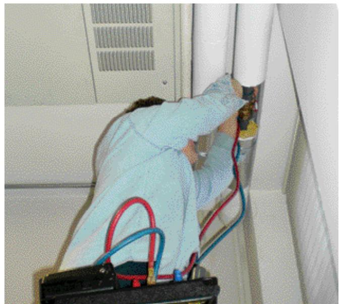
⚡ **TAB technician measuring water flow through a circuit setter.**
