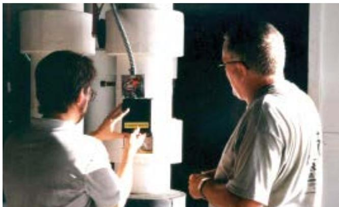
⚡ Technicians verifying the correct operation of a chilled water control valve.
