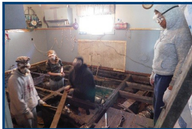
Working together to replace floorboards
