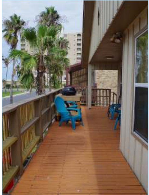
front deck spans width of house
