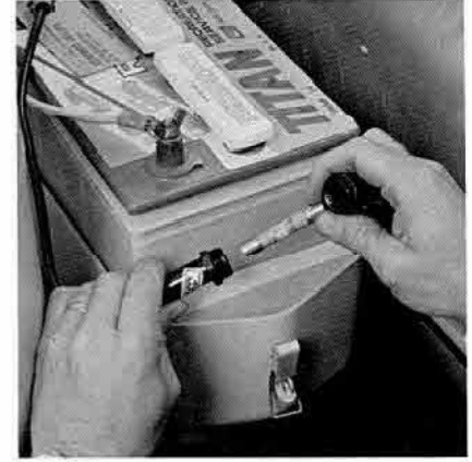
Battery In-Line Fuse
