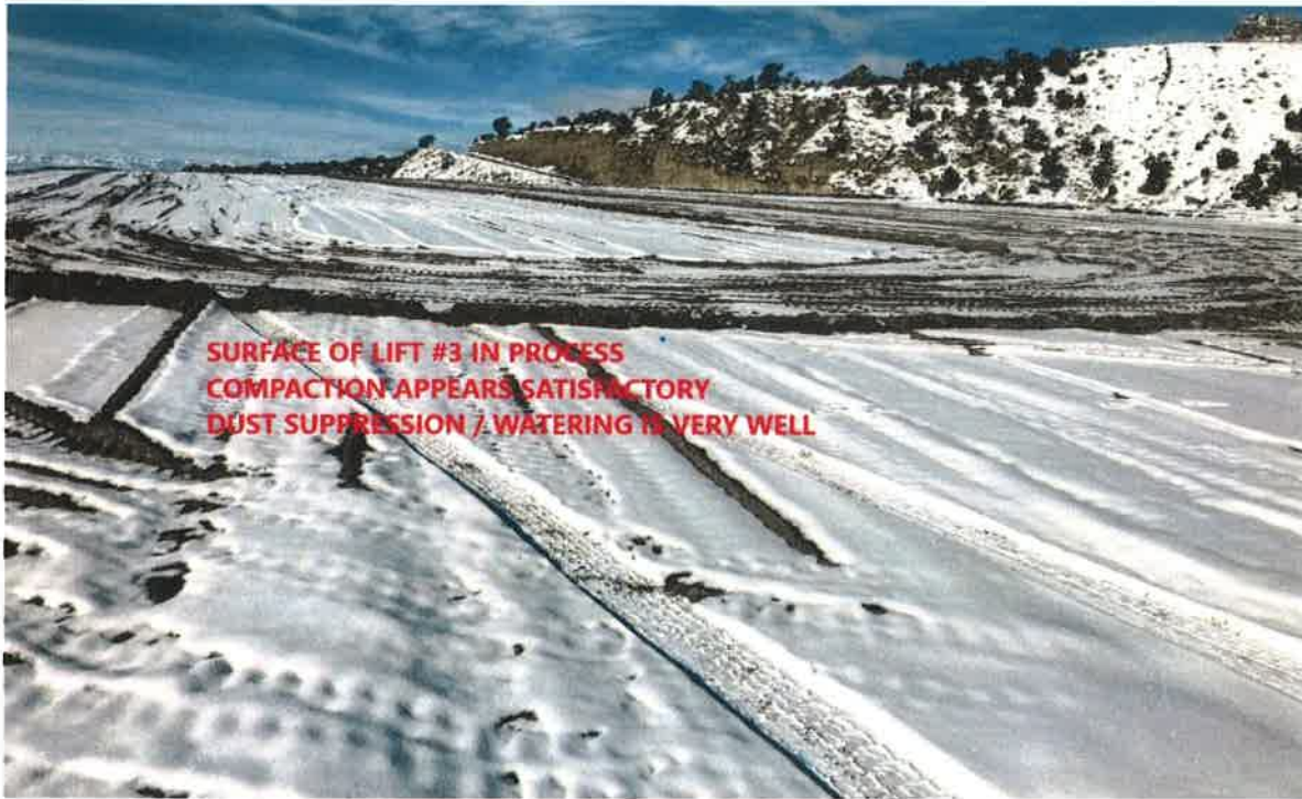
Surface of Lift #3 in process – photo looking northwesterly
