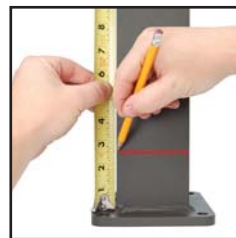
Measure up 2-1/2" from top of base plate
