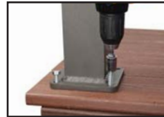
Fasten Post to Deck Surface
