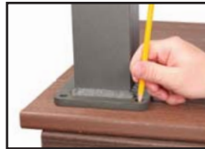
Mark and Pre-drill Holes
