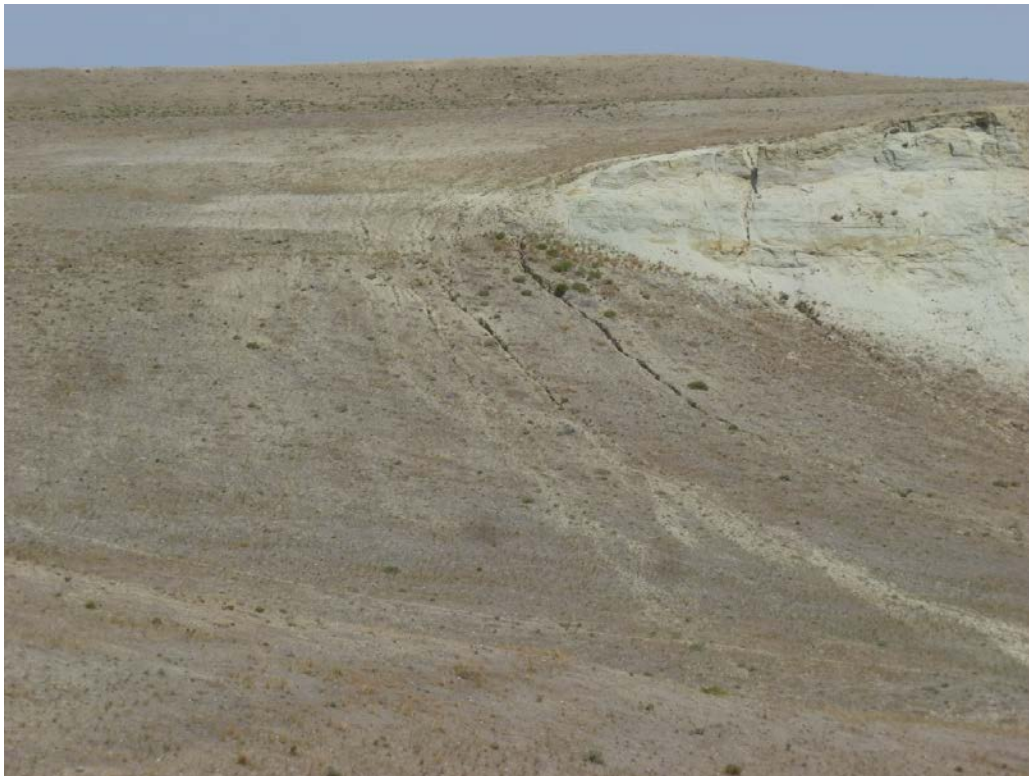
Photo 2. Minor erosion of recontoured and reclaimed area near the northeast end of high wall.
