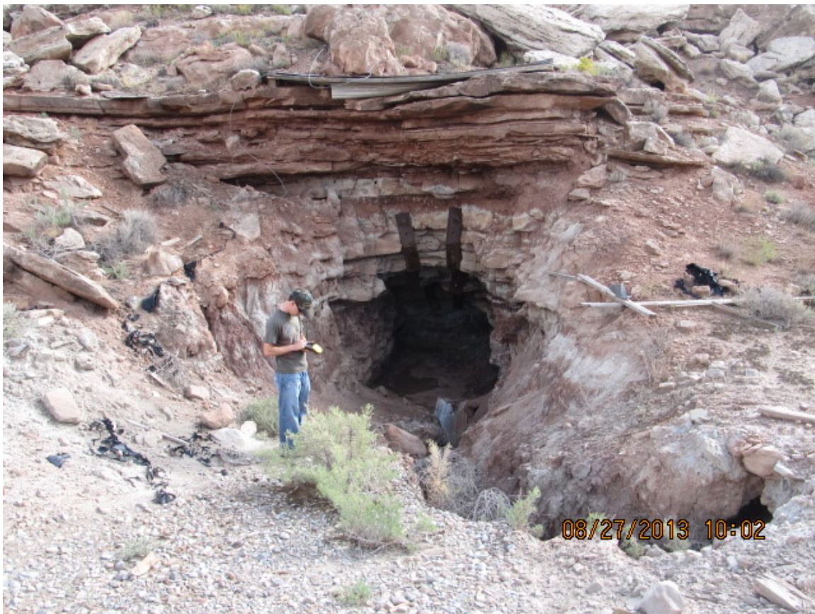
Figure 15. Yellow Cat District, Utah—Unstable, Unprotected Mine Opening
