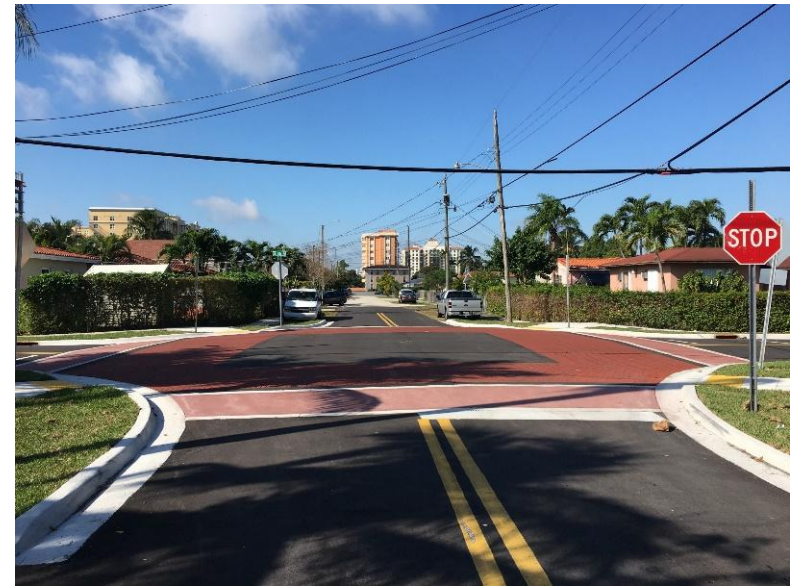
Raised Intersection with Textured Pavement (SW 36 th Avenue at SW 14 th Street)
