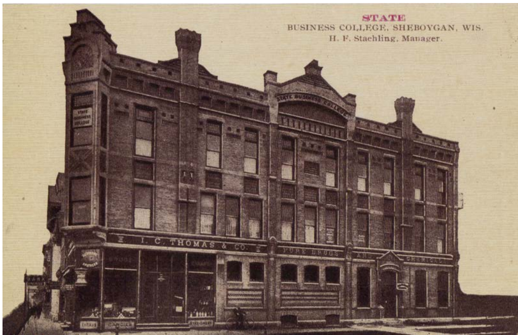
On April 11, 1887, the newly formed State Business College held its first class on the third floor of the new Zaegel Building on the southwest corner of North 8th Street and New York Avenue in Sheboygan. It was here that many Volga Germans went to night school to learn English.
