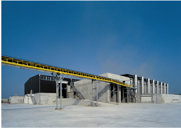
FIGURE 1. A bio-tunnel facility
