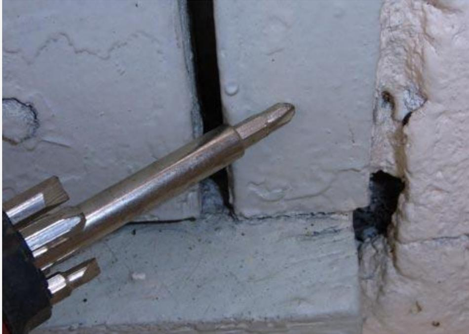
Above – A screwdriver comes handy in termite inspection. It is often used to tap wooden structures to determine hollow areas.
