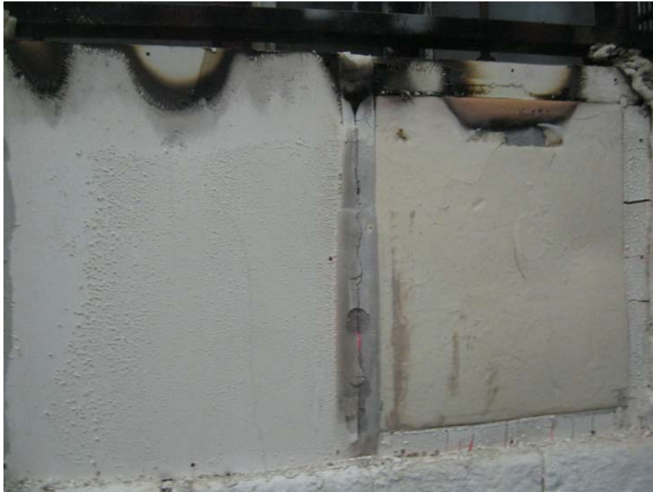
Test #3 - Exposed Side After the Fire Test
