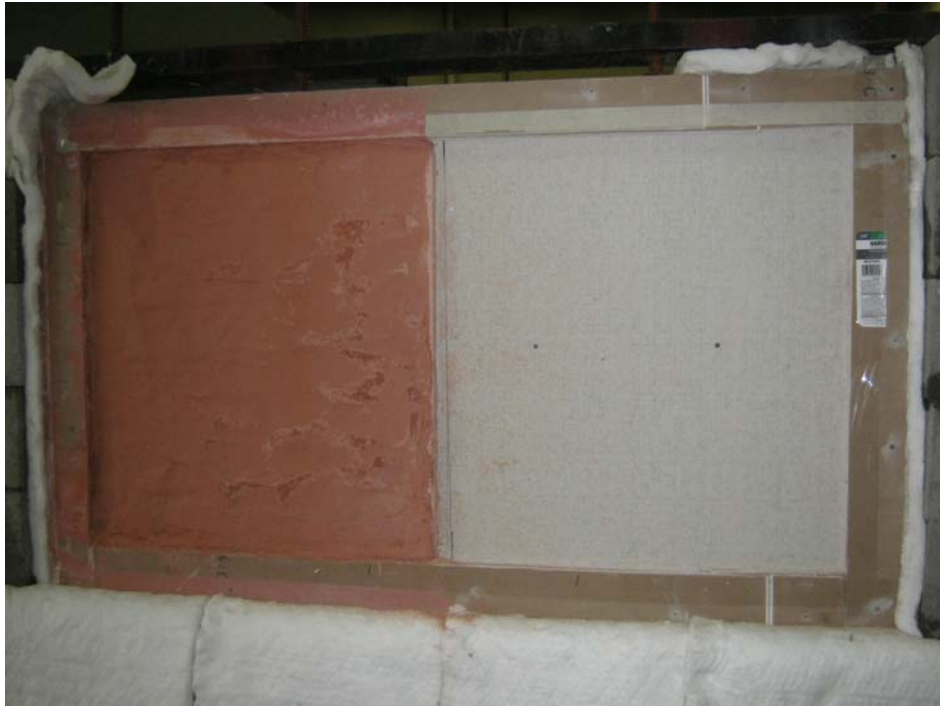
Test #1 - Exposed Side Prior to the Fire Test (FRC Left / Cement Board Right)
