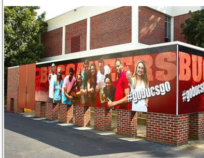
TS32- Frames on a Corner Wall. Printed graphics fixed and stretched on the side.
