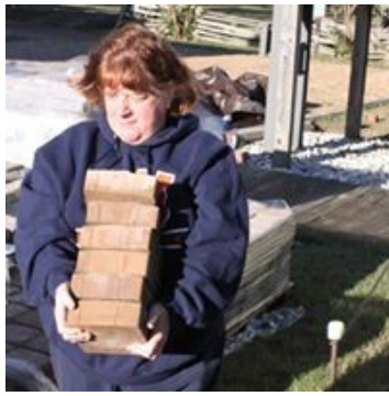
Everyone pitched in! Donna Fulk (photographer's better half) must have carried at least half of those pavers!
