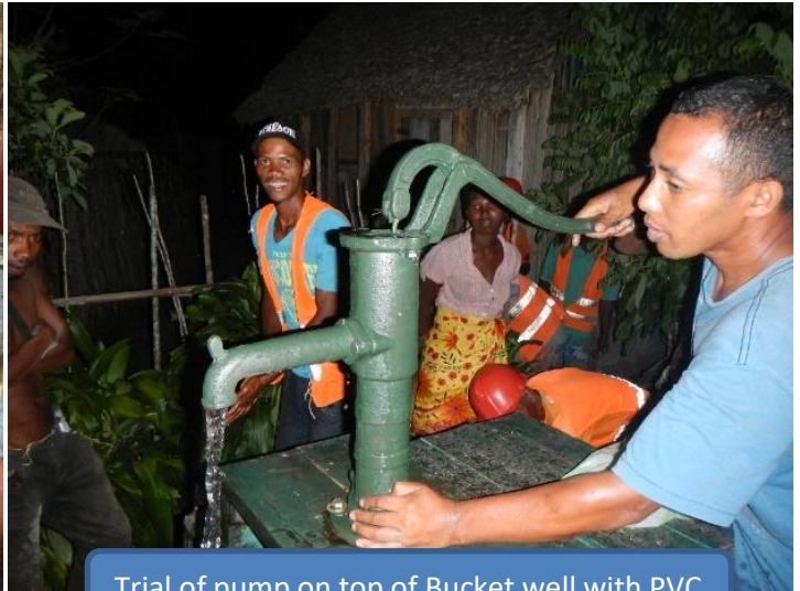
Trial of pump on top of Bucket well with PVC
