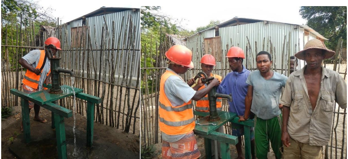
Pump working well, replaced leather cup
