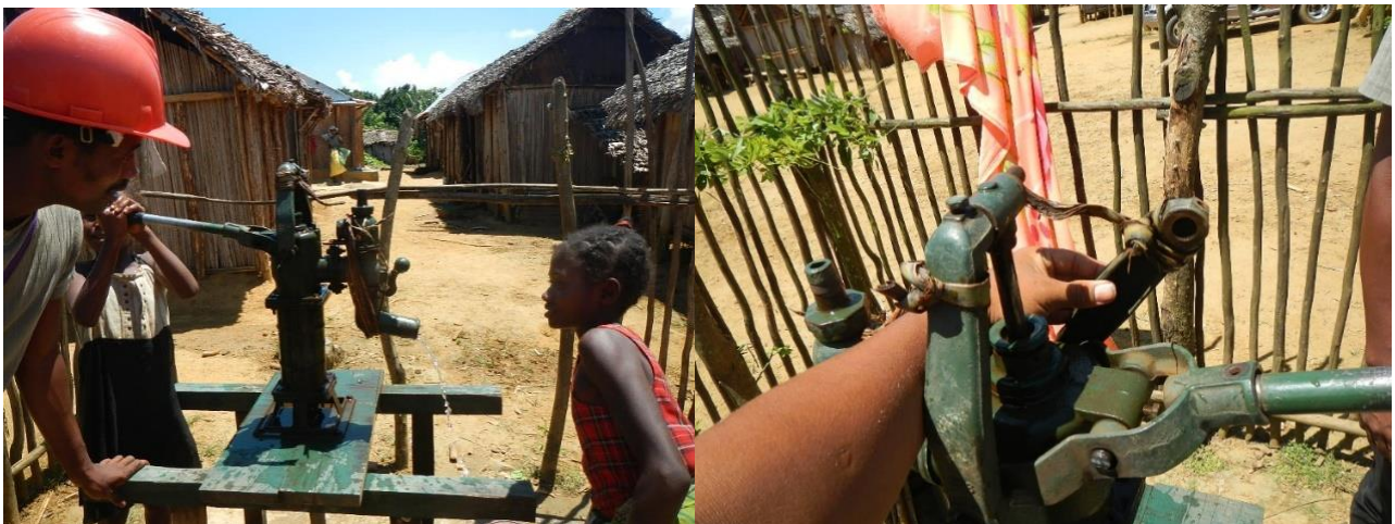
pump was working at very low flow, all was unscrewed, village tried to tighten it by using rope
