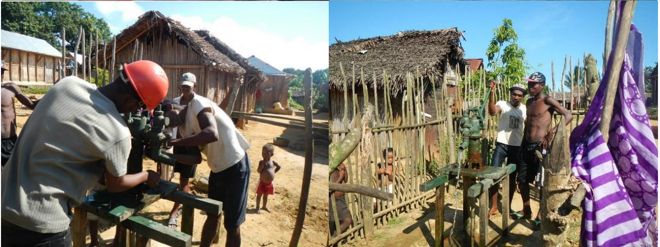
Pump was changed with the 20m pump from Tsivangiana, working well now
