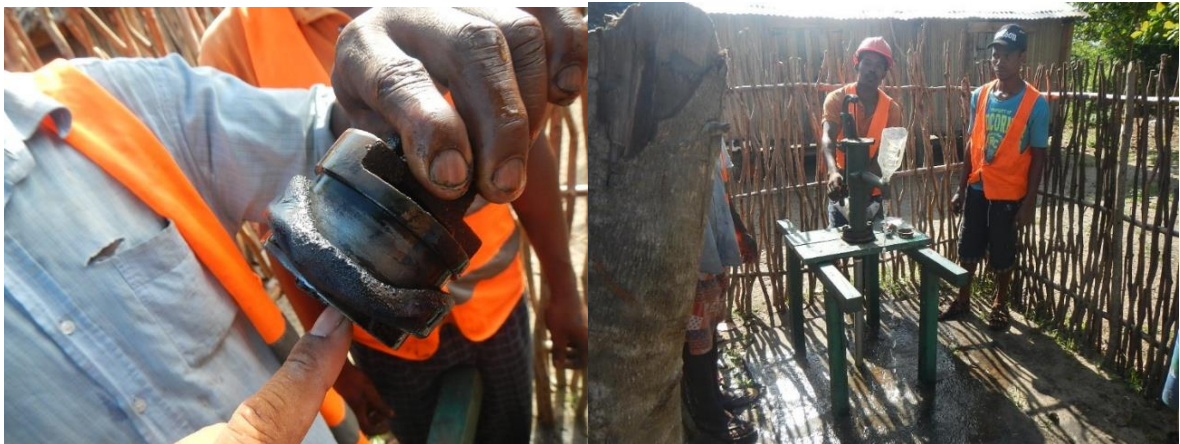
Pump was working but leather cup was worn, cup changed, working well
