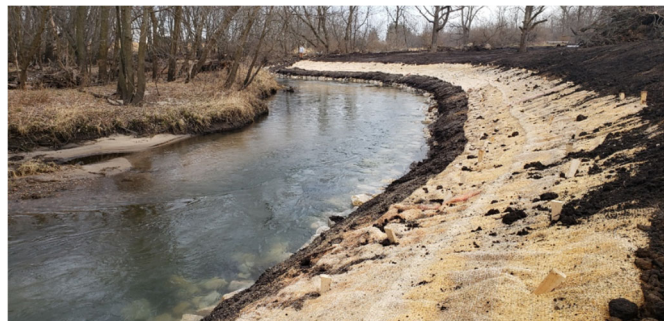
Streambank stabilization
