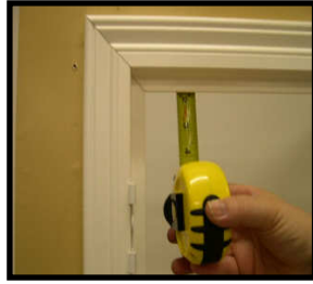
Measure Right & Top frame for spacing.
