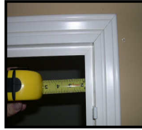
Measure Left & Top frame for spacing.
