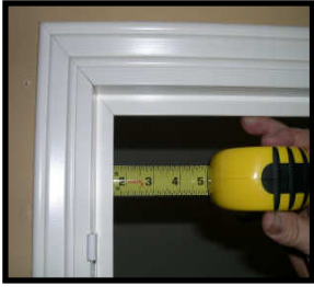
Measure Right & Top frame for spacing.
