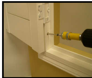
Pre-Drill bottom right & left frame.
