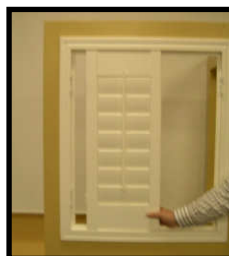
Position panel in the frame.
