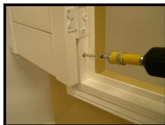
Only secure one screw into the bottom right frame.
