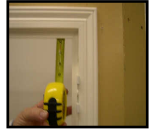
Measure Left & Top frame for spacing.
