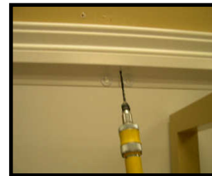
Pre-Drill middle of top and bottom frame.
