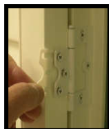
Insert spacer behind hinge.
