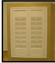
Slide panel into frame hinges and close other panel to hold in place.
