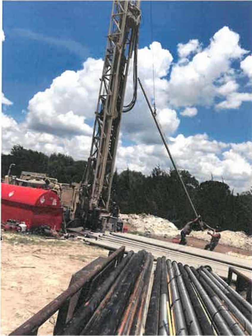
Red River Groundwater District Water Well Construction Photo
