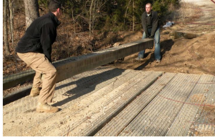
Above: Soldiers from EBOLC load normal balk from the M4T6 bridge.
